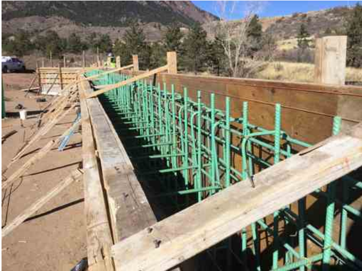
Placement of rebar for Abutment 1
