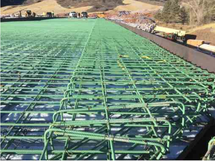
Bend section placement for sidewalk
