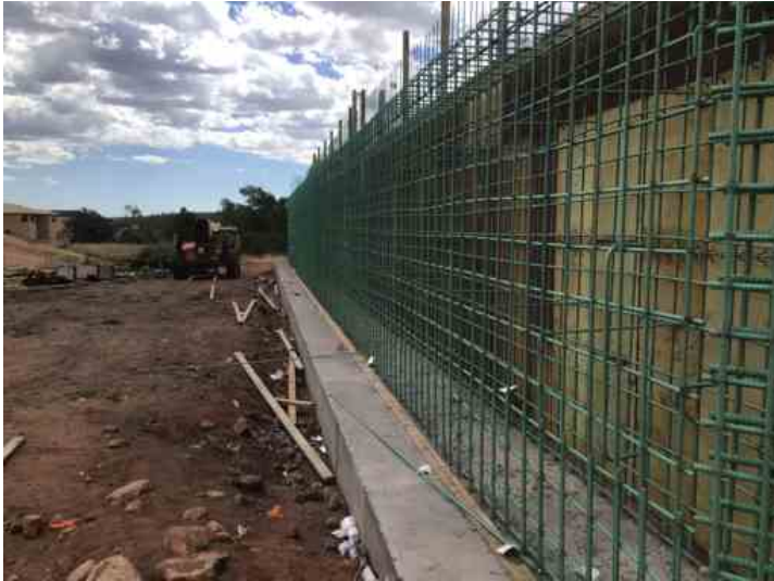
West abutment rebar
