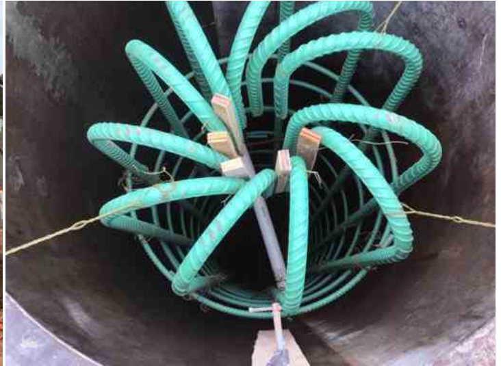
Column 6 reinforcement
