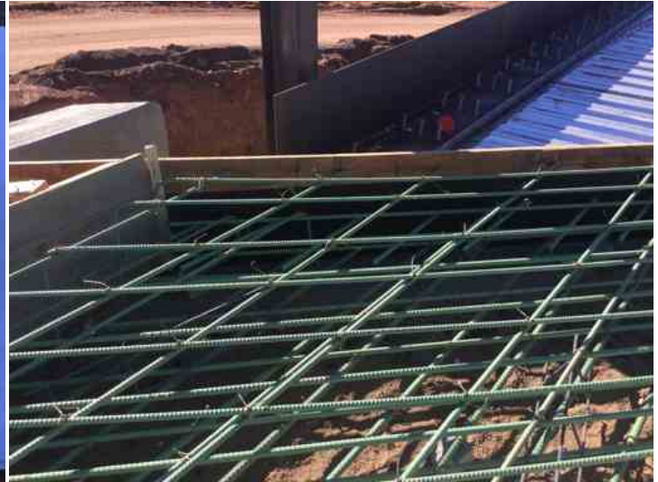
Bars out of clearance, touching the form.
