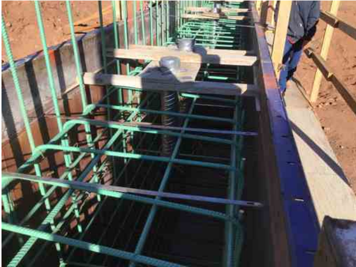
Rebar cage and embeds
