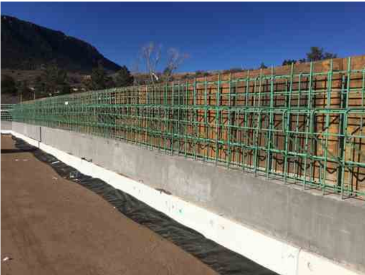
Partial completion of abutment 1, inner forms were not yet in place.
