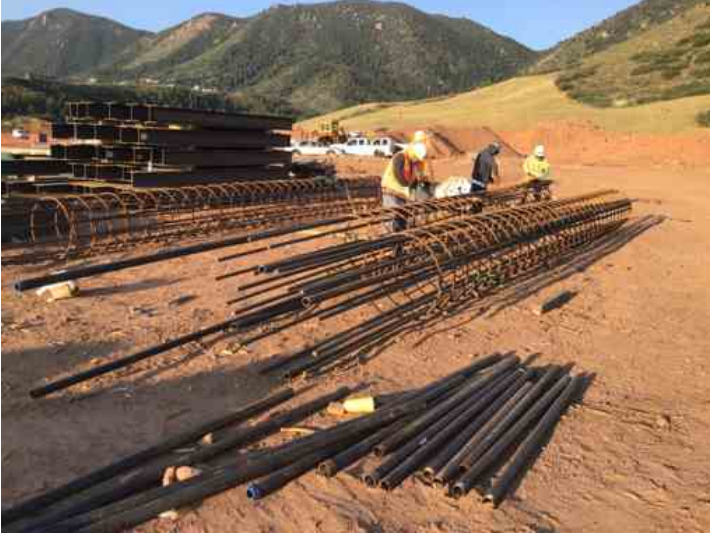
Rebar cage preparation
