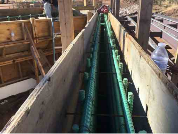
Reinforcement installed in Wingwall 3B
