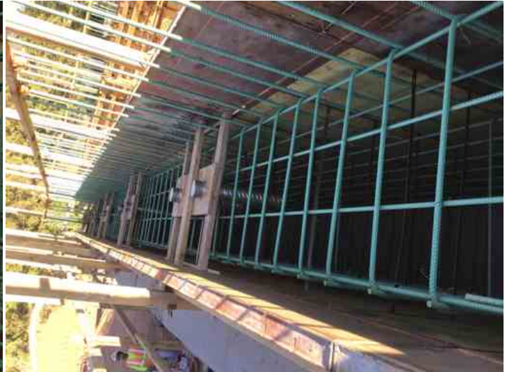
East abutment forms and embedded anchor bolts
