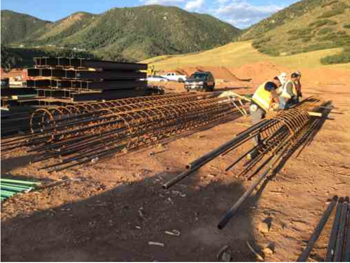
Reinforcement for caissons
