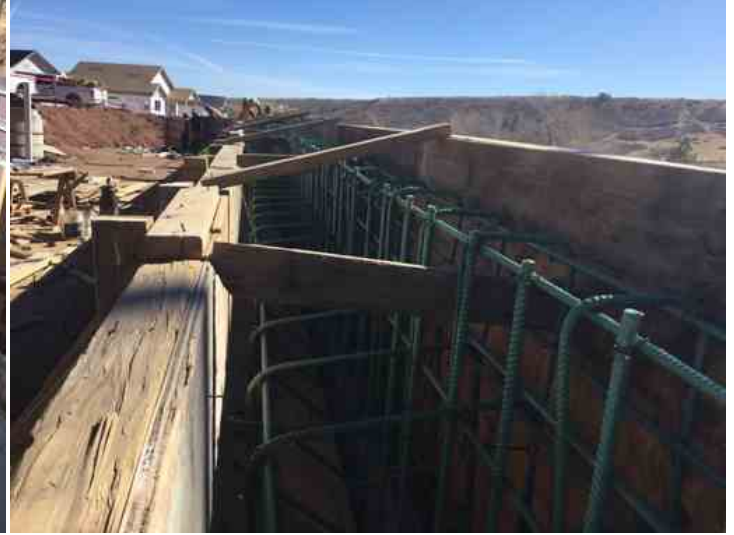
Reinforcement placement in abutment 3
