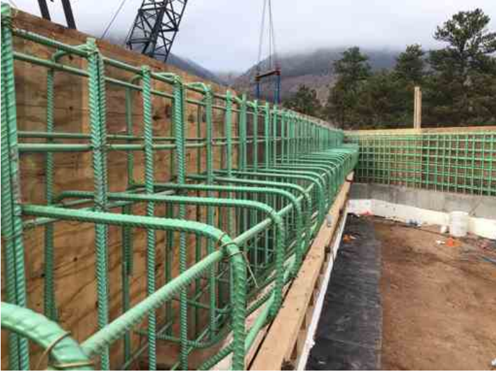
Abutment 3 rebar
