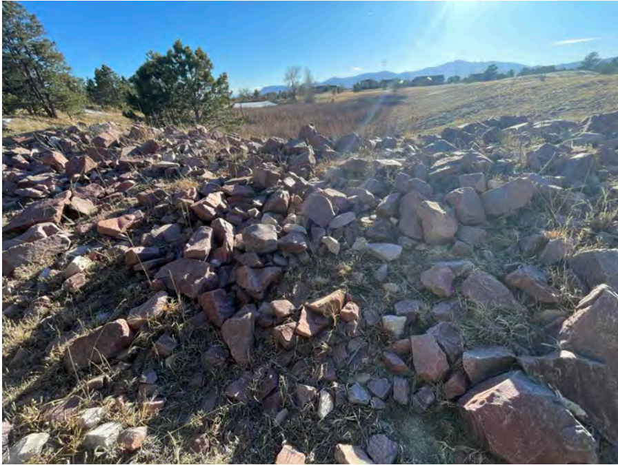
Pond 2 Emergency Spillway Looking downstream (southwest)
