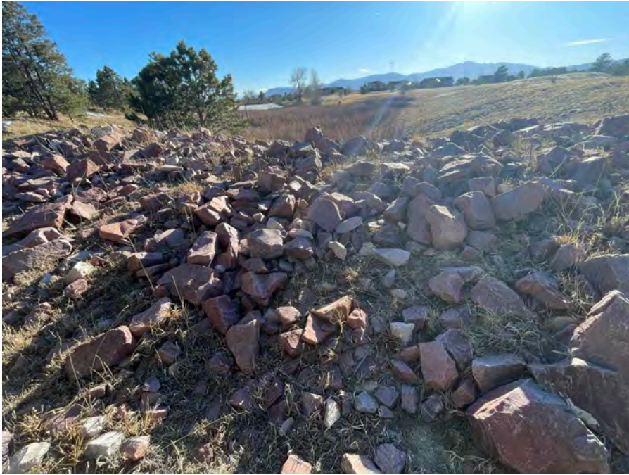
Pond 2 Emergency Spillway Looking downstream (southwest)
