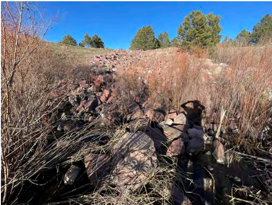
Pond 2 Emergency Spillway Looking upstream (northeast)
