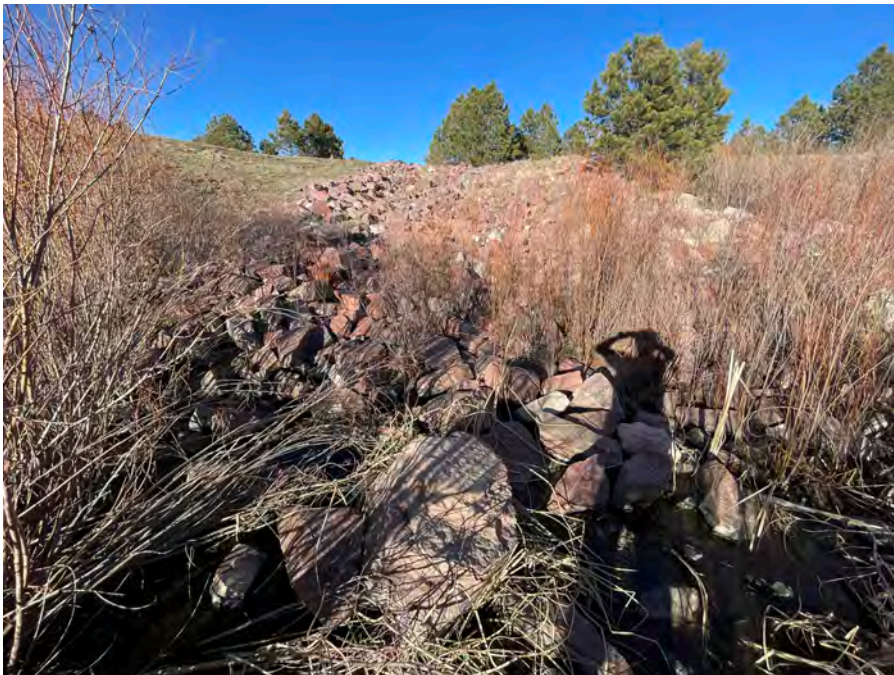
Pond 2 Emergency Spillway Looking upstream (northeast)
