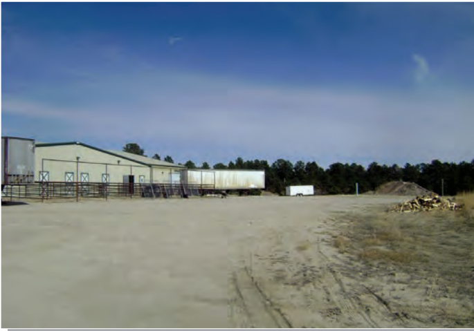
Photo 8a - Disturbed uplands and barn in the project area. View is to the northeast.
