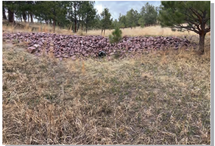
Photo 5b - Vegetated swale upstream of Cottonwood Creek in the project area. View is to the northwest.
