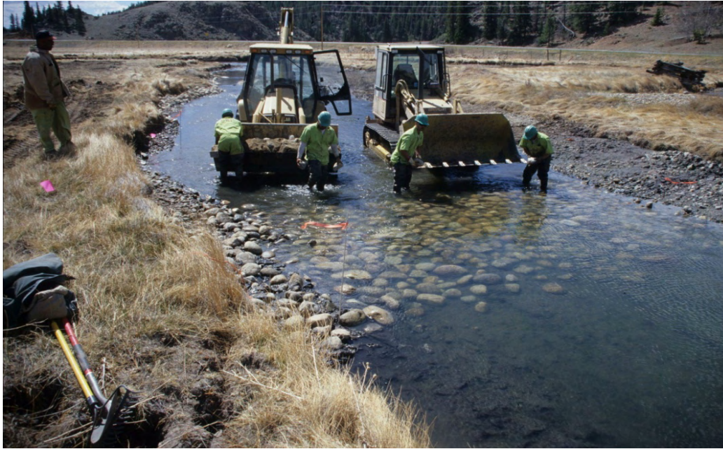
Figure A.2. Elevating riffle substrate.
