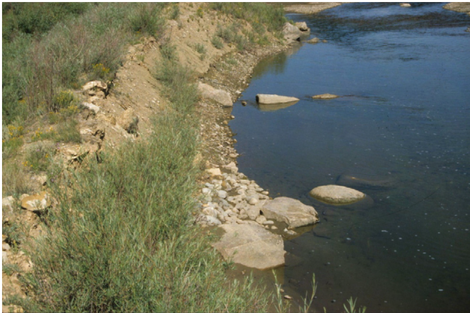
Figure A.15. Half cross (boulder) vane.
