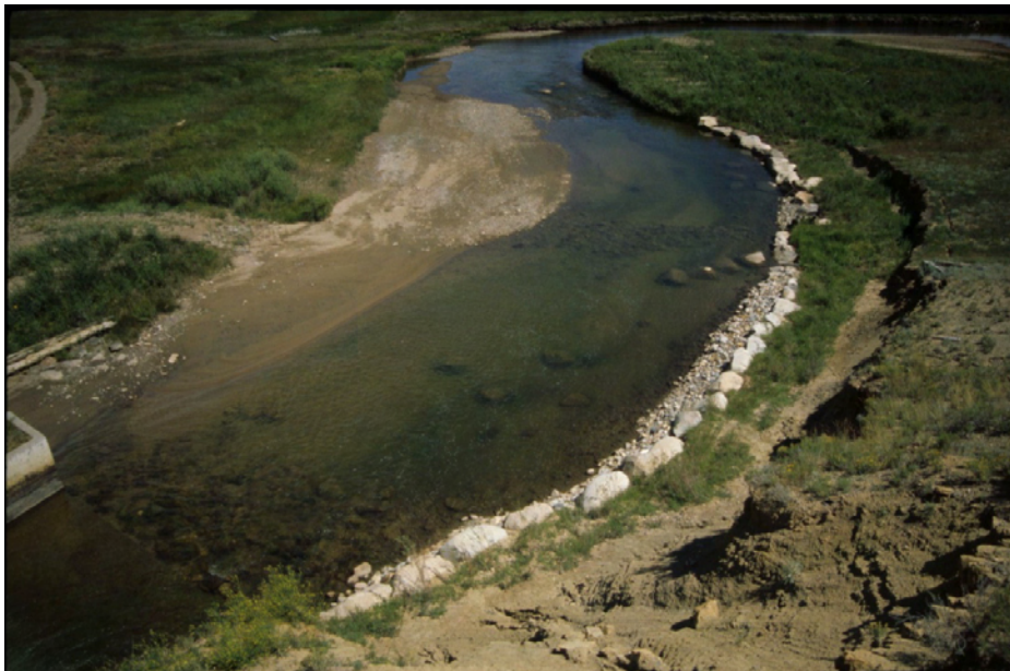
Figure A.9. Add a riparian bench with a stone/boulder toe.
