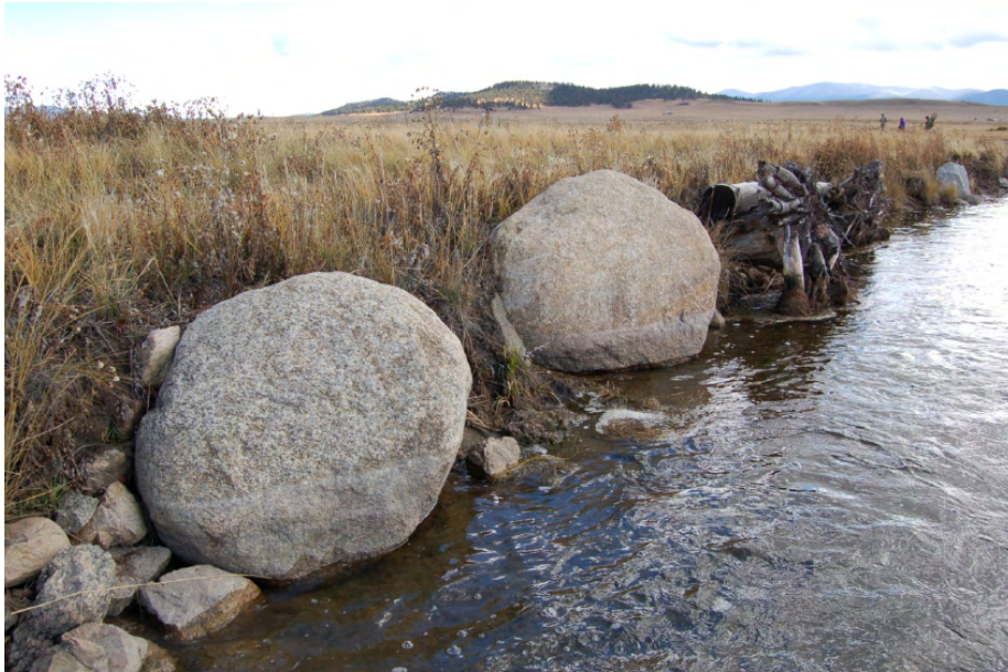
Figure A.18. Single boulder deflector.
