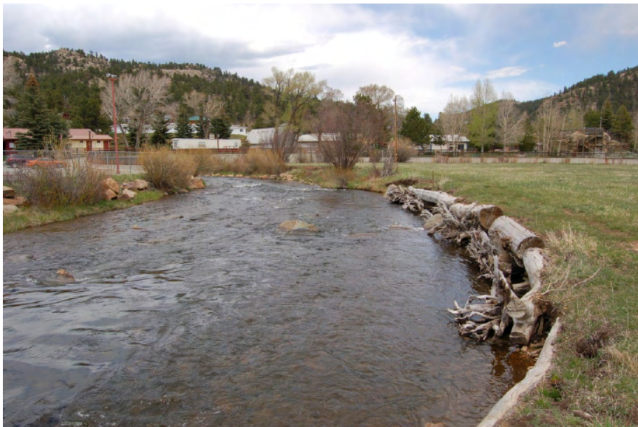
Figure A.13. Horizontal parallel log.
