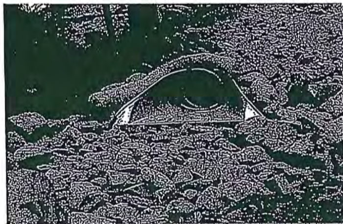
Photograph TOP-1. Riprap outlet protection.
