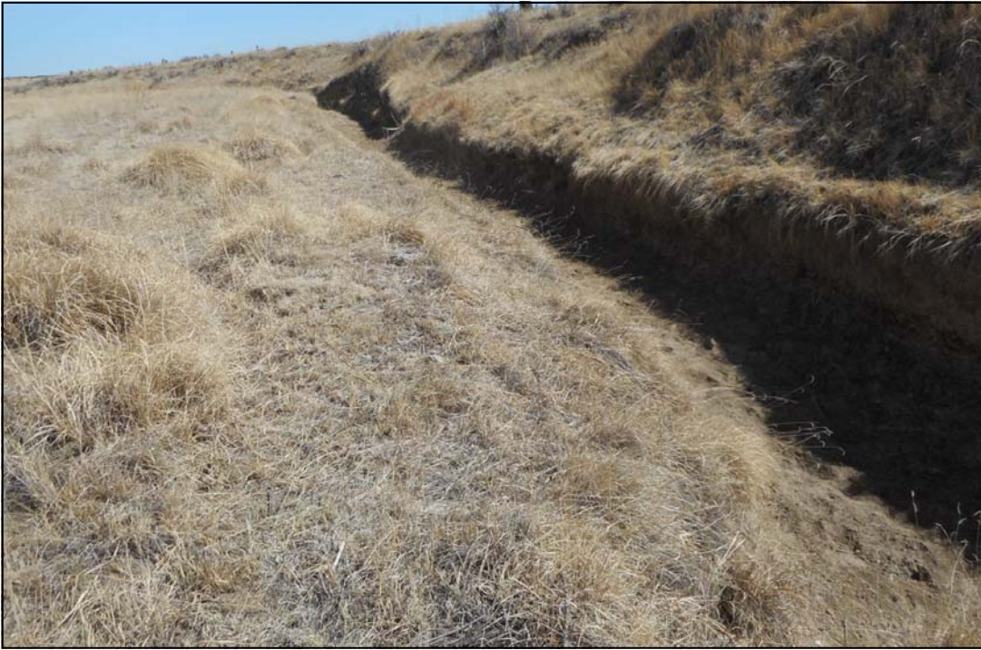
Photo 3. Eroded channel of Williams Creek, looking upstream/north. 3-30-18
