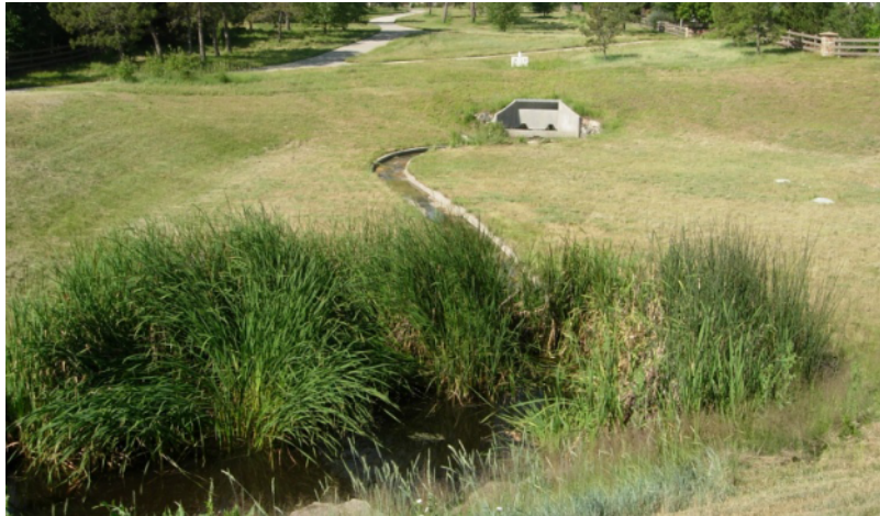
Figure 32. - Full Spectrum Extended Detention Basin
