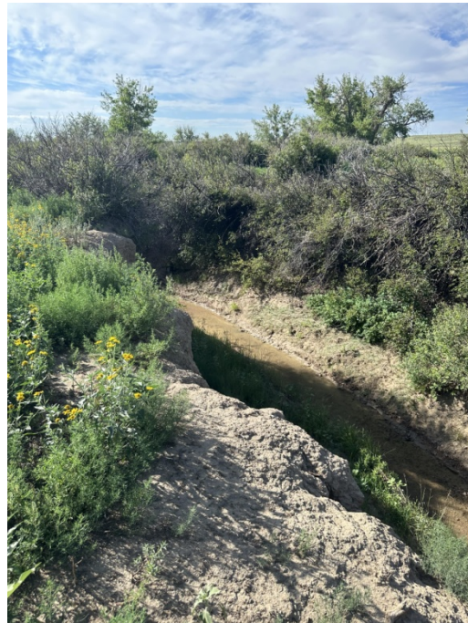
Figure 10. – Photo of Portion of Eroded Rock Creek Channel
