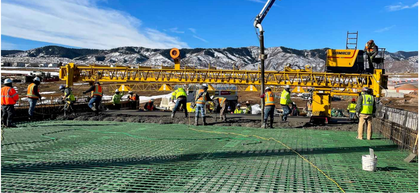
Figure 17. High Capacity Roadway Construction
