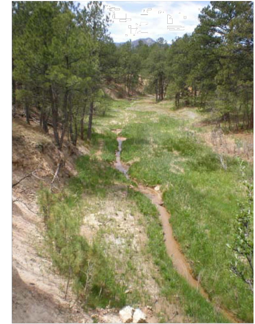
AFTER NATURAL CHANNEL CONSTRUCTION
