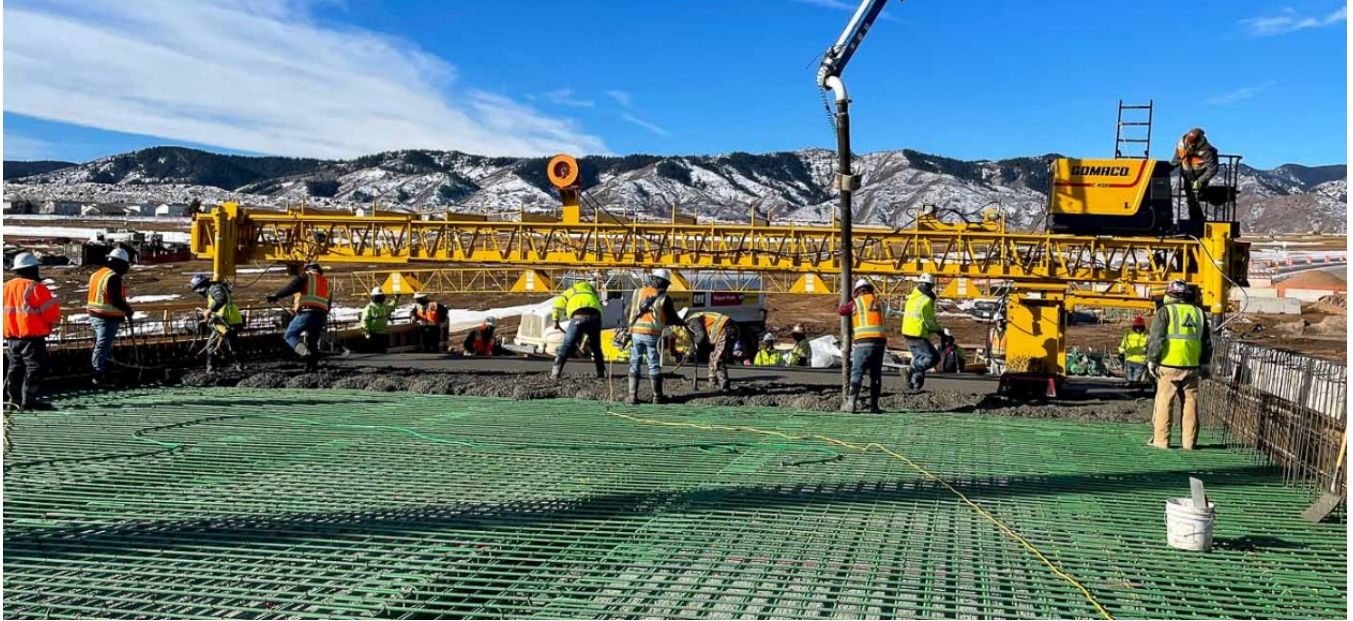
Figure 17. High Capacity Roadway Construction
