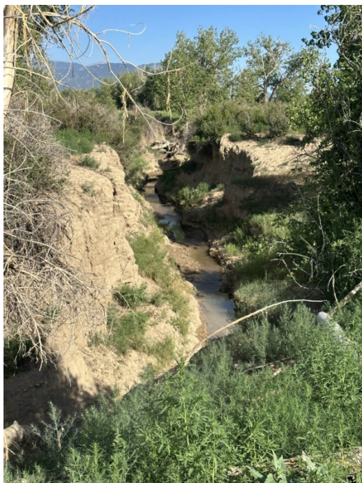
Figure 9. - Photo of Portion of Eroded LF Creek Channel
