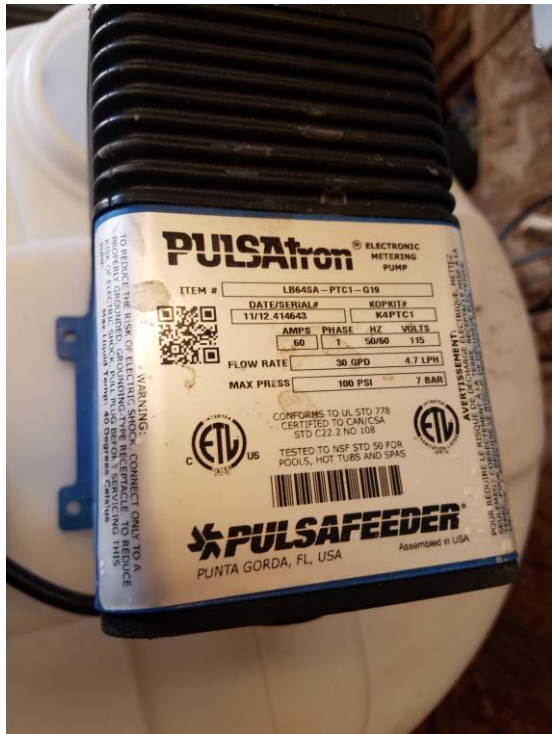
LFH2 Chlorine Pump Nameplate
