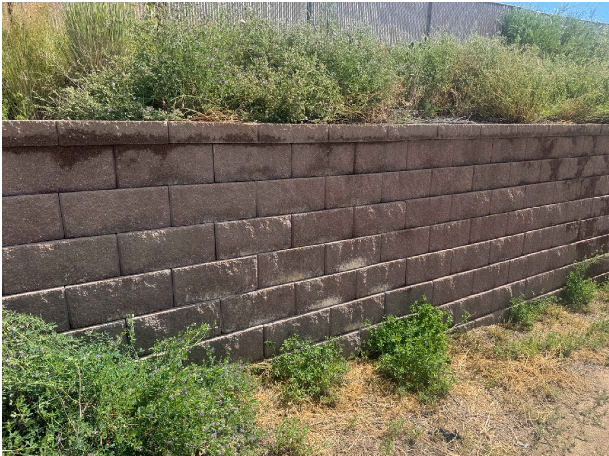
EXISTING MSE BLOCK RETAINING WALL PHOTO
