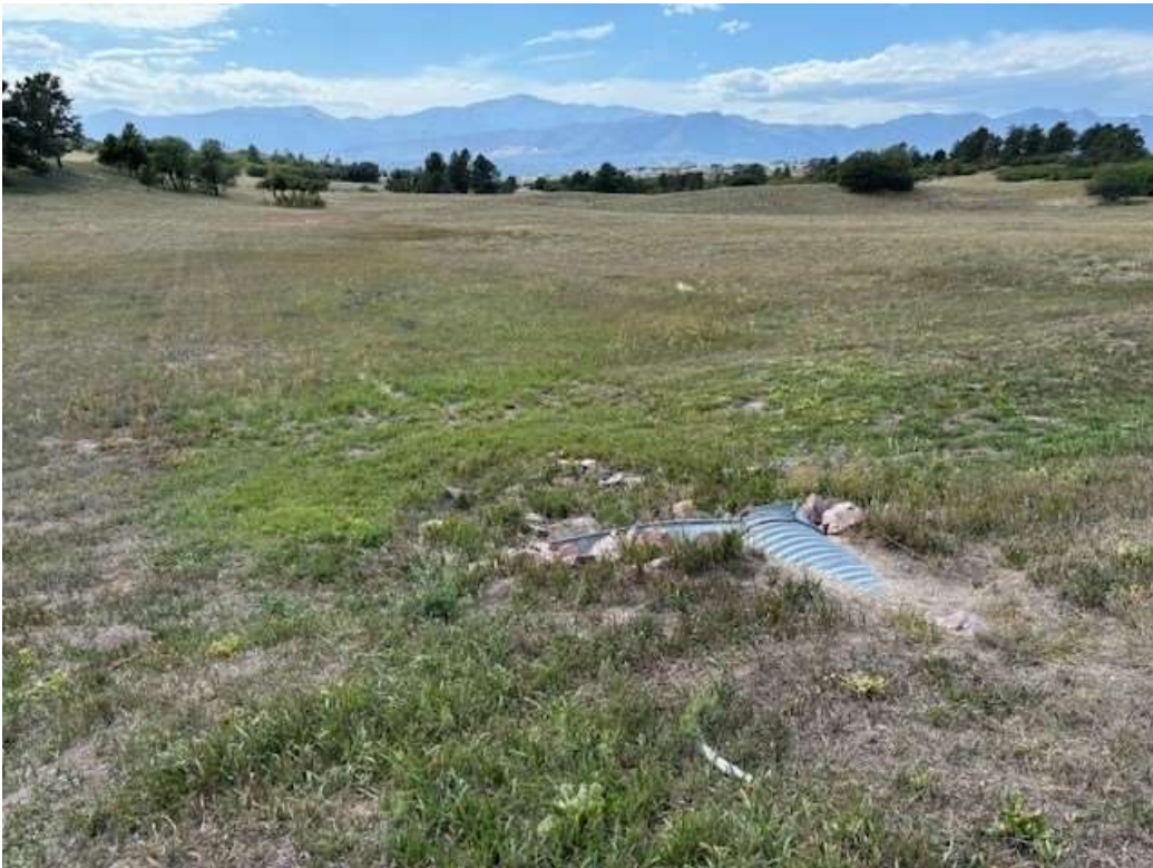
Existing Culvert Q – RR outlet apron and stable grass-lined channel downstream
