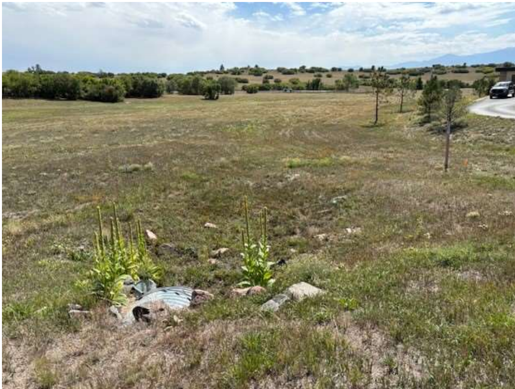
Existing Culvert P - RR outlet apron and stable grass-lined channel downstream
