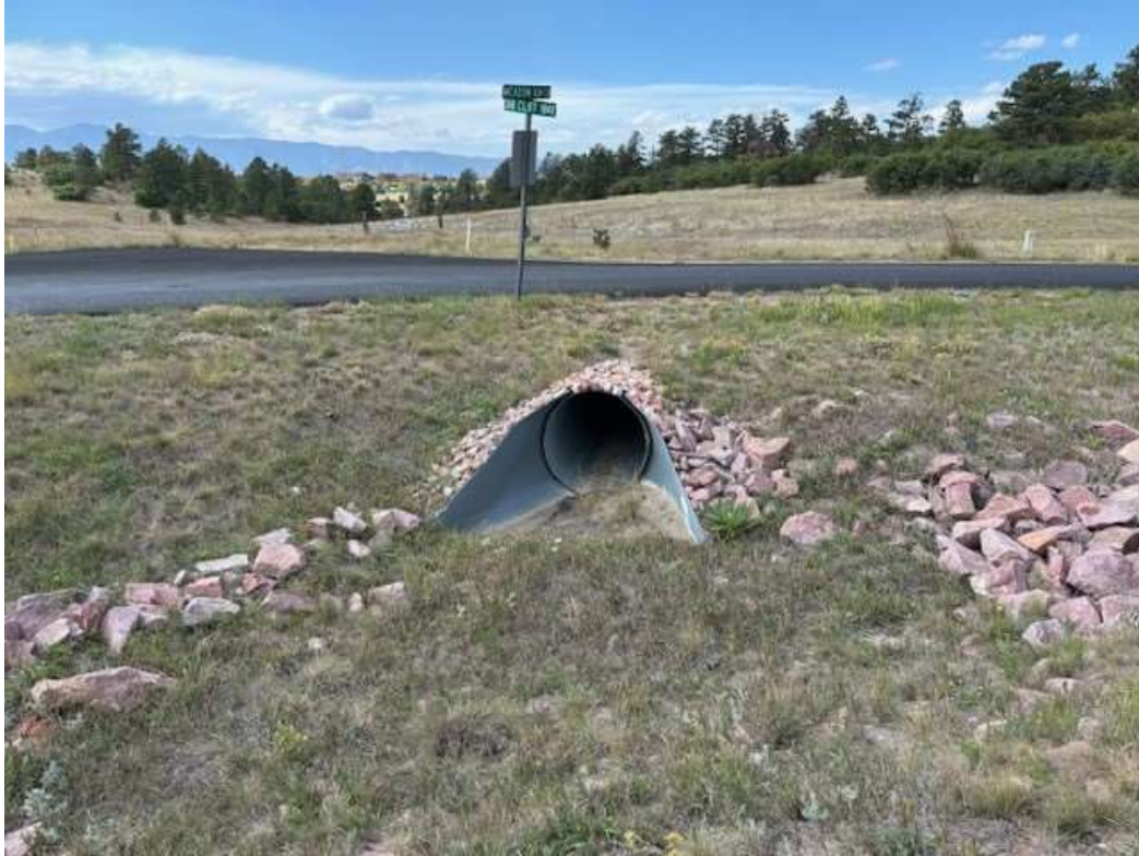
Existing Culvert K – 36” CMP Inlet with RR apron (facing west
