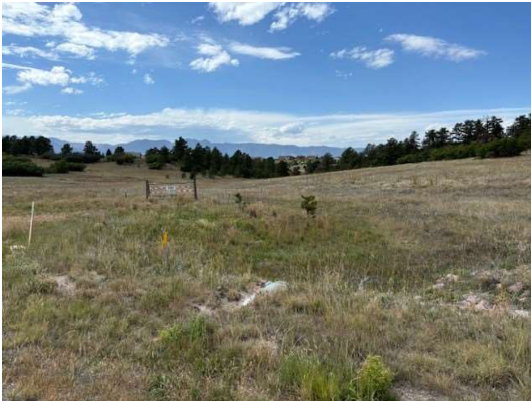
Existing Culvert K – RR outlet apron and stable grass-lined channel downstream
