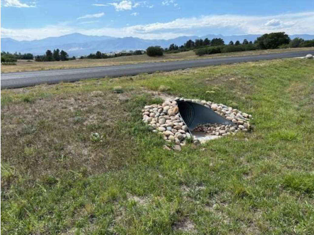
Existing Culvert Q – 30” CMP Inlet with RR apron (facing SW)
