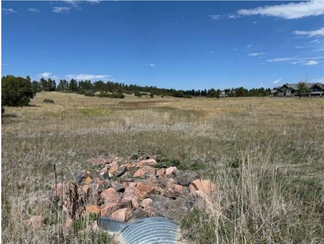
Existing Culvert P - 48" CMP Inlet with RR apron (facing NE; typical vegetation within Filing Three)
