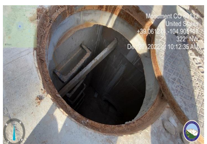
Photo 8: Remove forms from inlets along Mesa Top Dr North and Mesa Top Dr South
