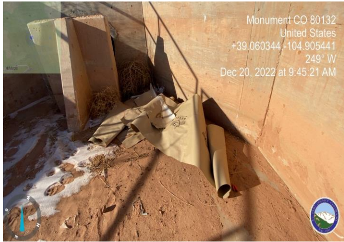
Photo 5: Remove sediment and debris from pond forebay
