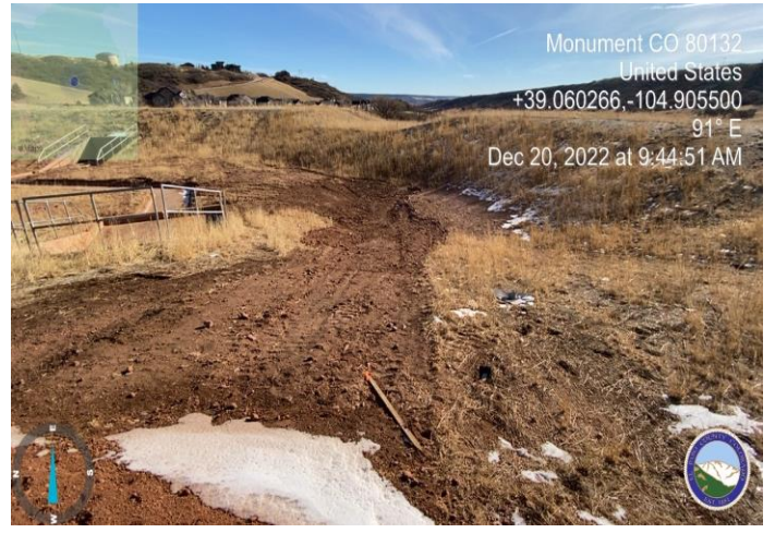
Photo 6: Stabilize and seed pond slopes and disturbed area (FA requirement, so just a reminder at this point)
