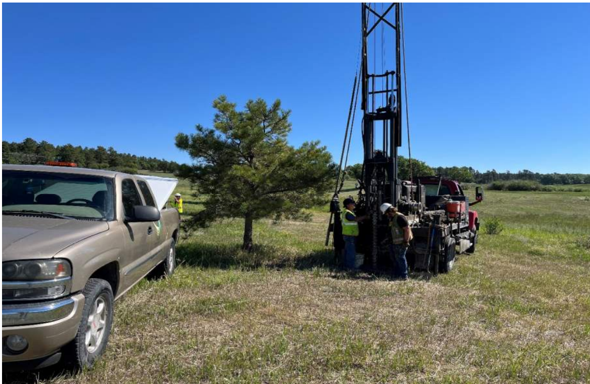
DRILLING BORING BH-2 - LOOKING NORTHEAST
