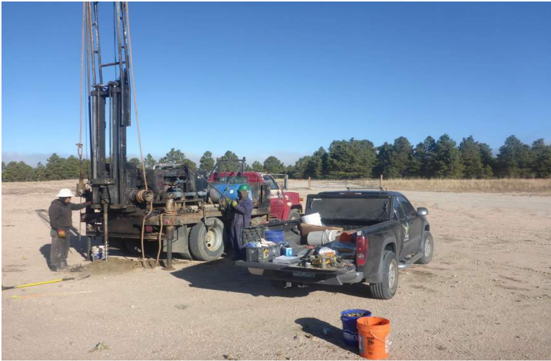
DRILLING BORING TK-4 - LOOKING NORTH
