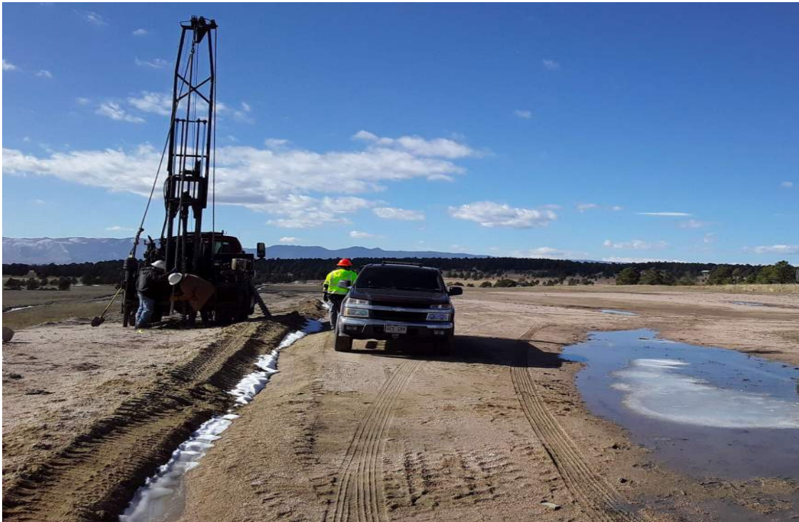
DRILLING BORING TK-5 - LOOKING WEST
