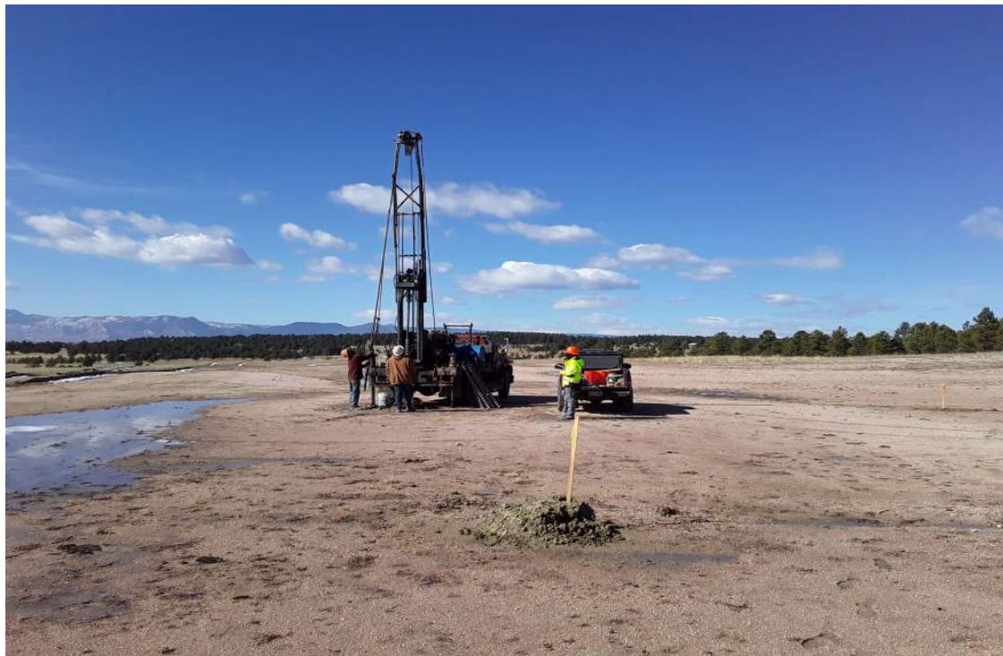
DRILLING BORING TK-3 - LOOKING WEST
