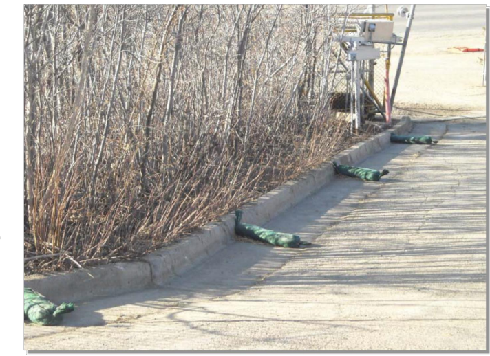
Photograph RS-1. Rock socks placed at regular intervals in a curb line can help reduce sediment loading to storm sewer inlets.
