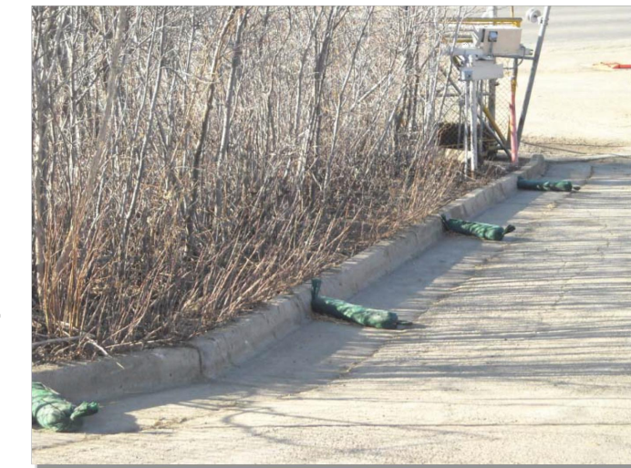
Photograph RS-1. Rock socks placed at regular intervals in a curb line can help reduce sediment loading to storm sewer inlets. Rock socks can also be used as perimeter controls.
