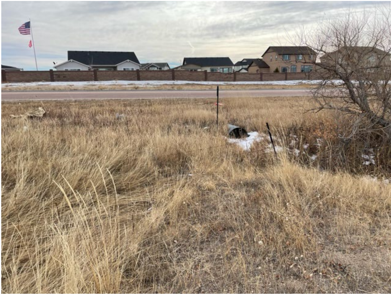
Photo 5. Looking southeast at a culvert under Vollmer Road.
