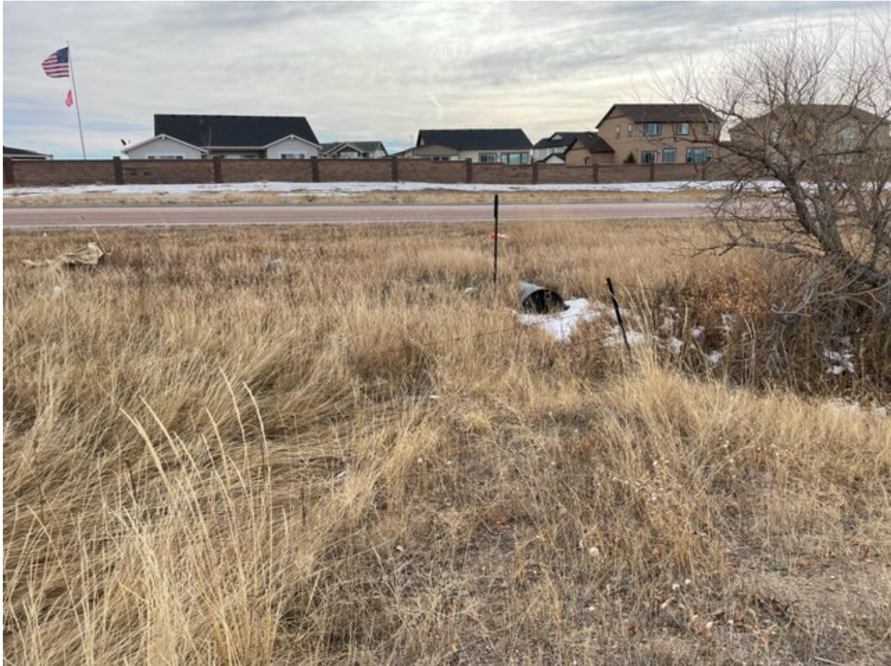
Photo Location 10. Looking southeast at culvert inlet directed offsite under Vollmer Road.
