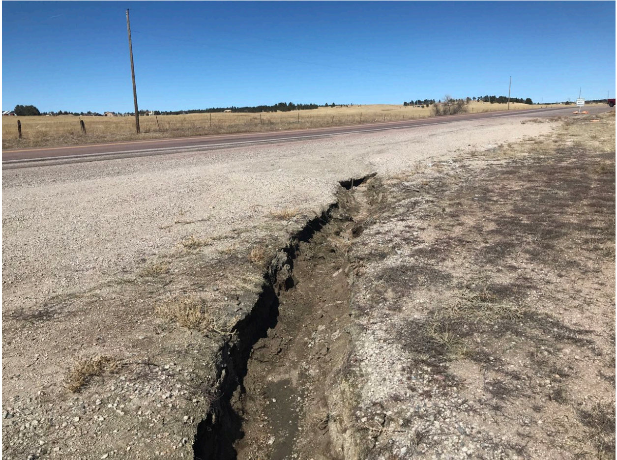
Photo Location 01. Looking northwest at drainage channel on east side of Vollmer Road.
