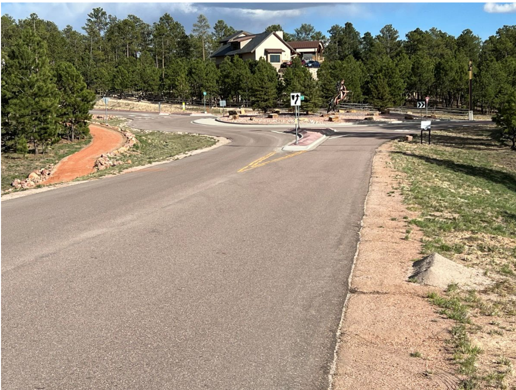
Photo Number: 5EP.10617_10 Description: Looking at the roadway as it approaches the roundabout with Shortwall Drive. The roadway turns to the left (north) where it ends at its eastern terminus, consisting of a roundabout at Stagecoach Road and Old Stagecoach Road. View: Southeast
