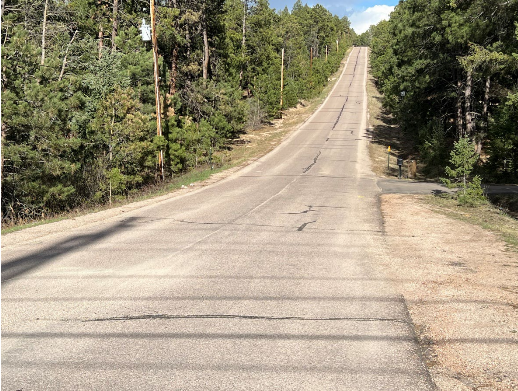
Photo Number: 5EP.10617_1 Description: Looking at the roadway as it traverses east from the western terminus, which is the intersection of Stagecoach Road and Roller Coaster Road. Note the steep incline. View: East
