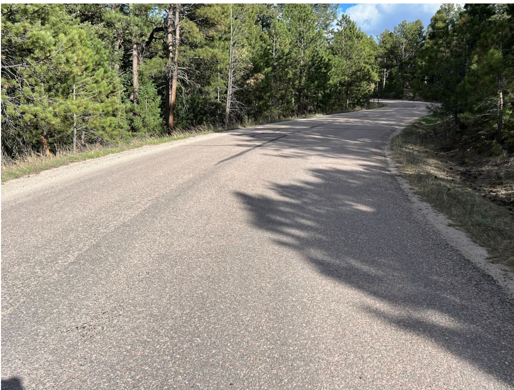
Photo Number: 5EP.10617_2 Description: Continuing east along the roadway. View: Southeast
