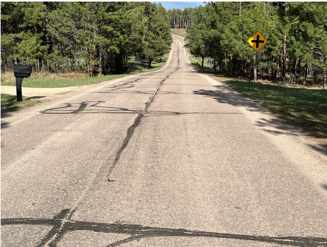
Photo Number: 5EP.10617_6 Description: Looking along the roadway as it approaches SH 83 in the distance. View: East
