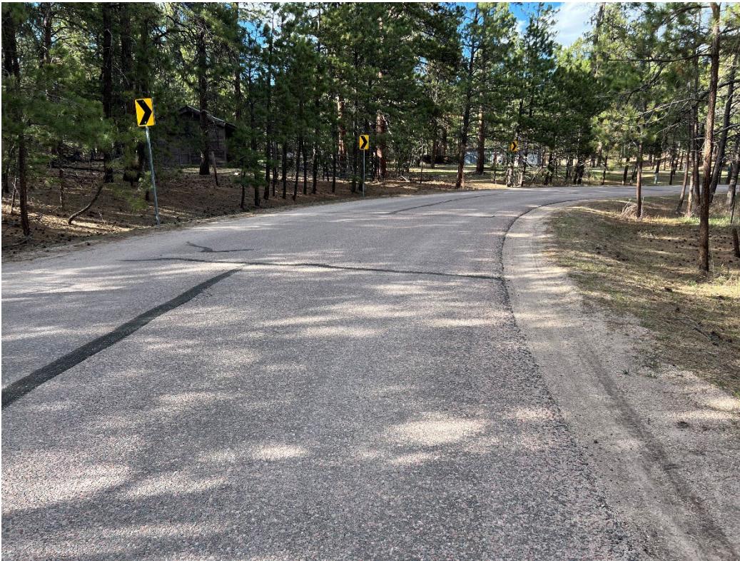
Photo Number: 5EP.10617_5 Description: Traversing east along the roadway. View: Northeast
