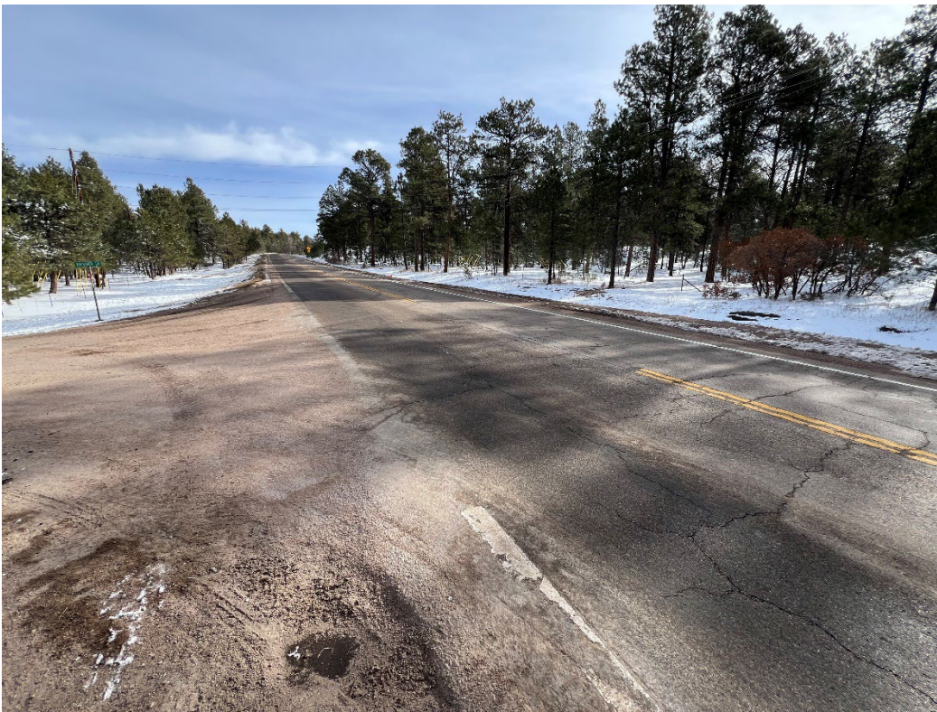
Photo Number: 5EP.7714.5_9 Description: View of the southern terminus of the segment, at the SH 83 and Kaessner Lane intersection. View: Northeast
