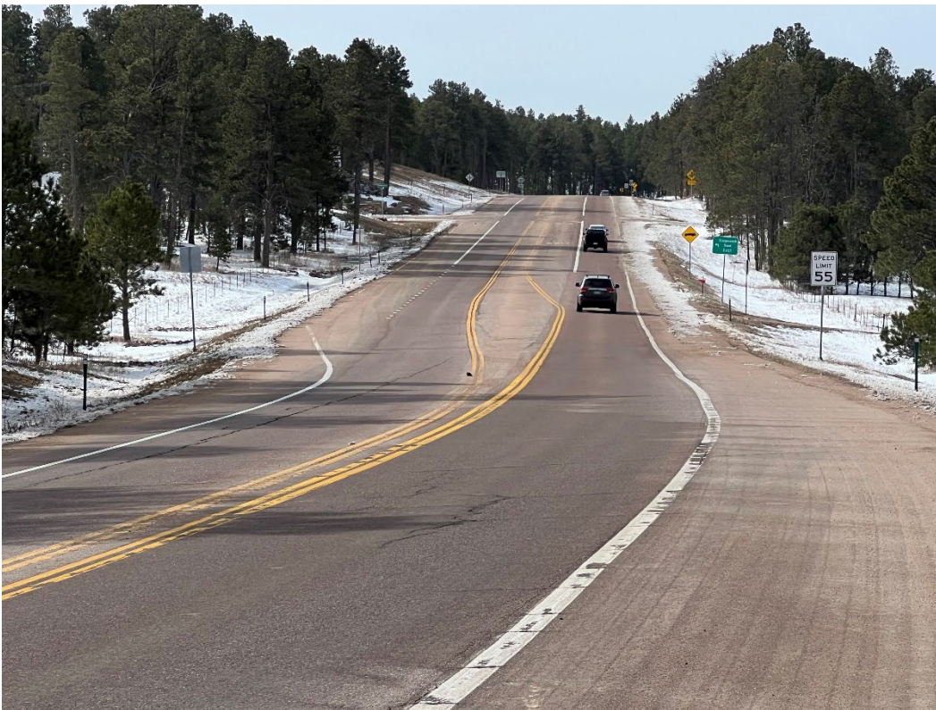
Photo Number: 5EP.7714.5_2 Description: Looking south along the segment.
