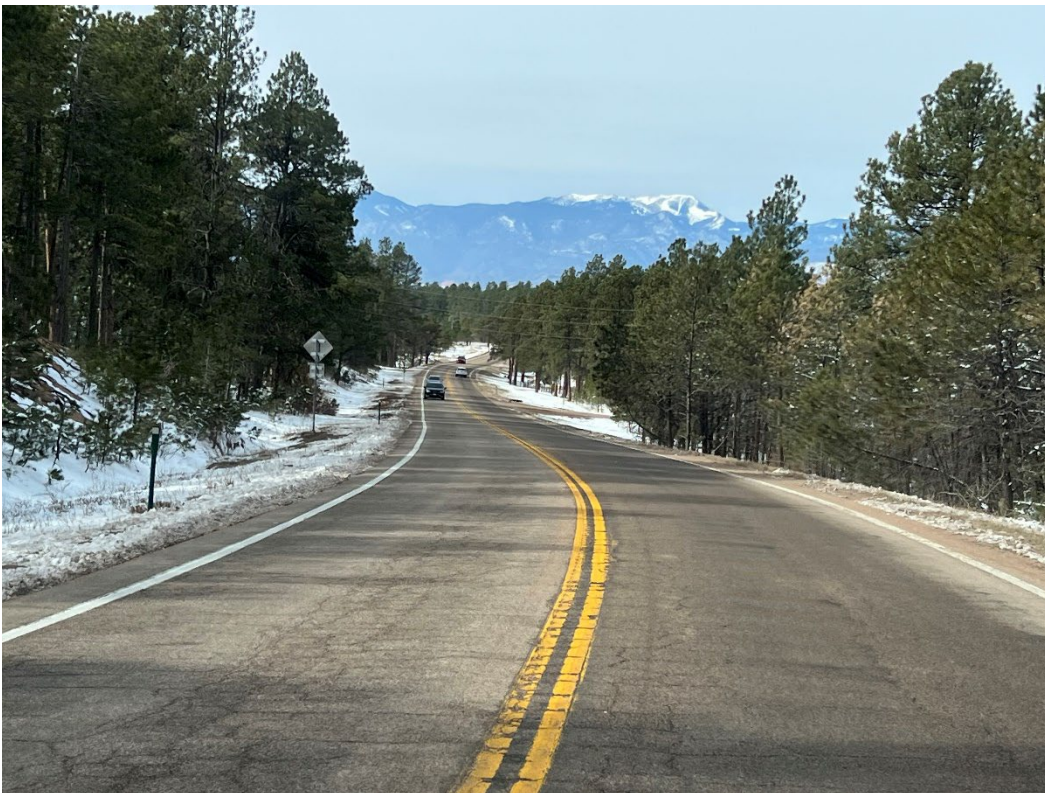
Photo Number: 5EP.7714.5_8 Description: Looking south as the segment approaches its southern terminus. View: South
