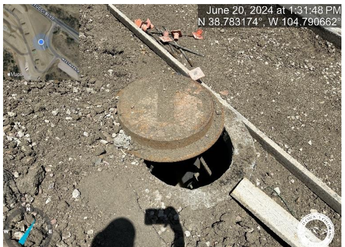
Photo 12: Clean out sediment from manhole.
