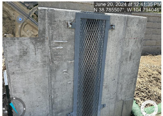
Photo 4: Install No. 93 Johnson Vee Wire stainless steel well screen.
