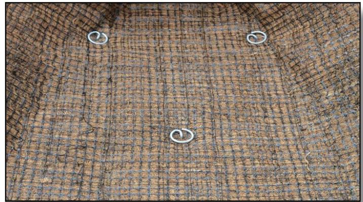
*VMax turf reinforcement mat being installed on a channel application (top right), twist pins installed with TRMs can have increased system performance and pullout resistance (middle right), twist pins are available in 8" and 12" lengths and two coil configurations designed for hard or soft soil types (lower right).*
