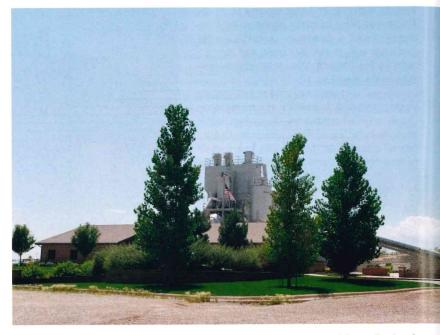
Powered partly by wind-derived energy from Black Hills Power turbines, the batch plant is designed to sit below grade from one side and placed behind a larger office structure to further reduce surrounding area impact. Pete Lien & Sons team members plant upward of 1,000 trees annually in a nearby area.
