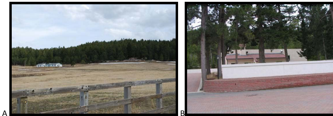
Figure 25: A few of the structures found on the property. (A) The parsonage as viewed from the main gate and (B) the church as viewed from the north.
