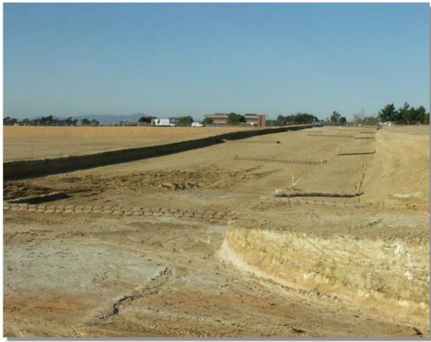
Photograph RCS-1. Rough cut street controls.
