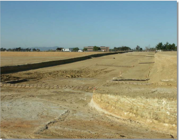
Photograph RCS-1. Rough cut street controls.
