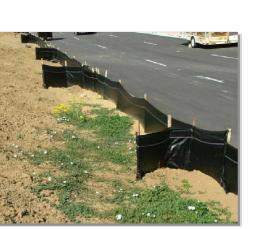
**Photograph SF-2.** When silt fence is not installed along the contour, a "J-hook" installation may be appropriate to ensure that the BMP does not create concentrated flow parallel to the silt fence. Photo courtesy of Tom
