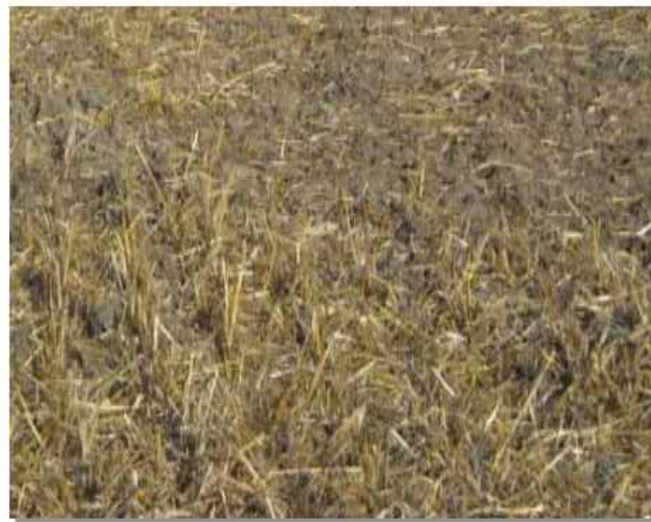
Photograph MU-4. An area that was recently seeded, mulched, and crimped.
