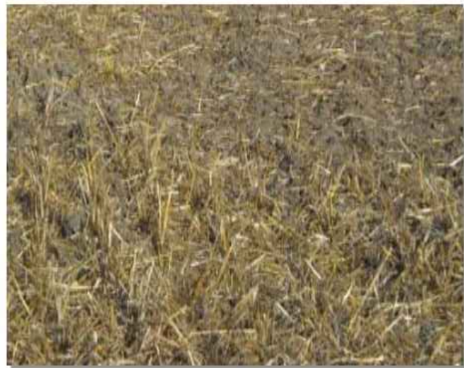
Photograph MU-4. An area that was recently seeded, mulched, and crimped.
