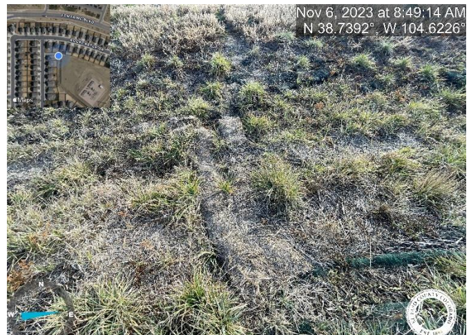
Photo 16: Substation Swale 2: Remove temporary control measures from swale.
