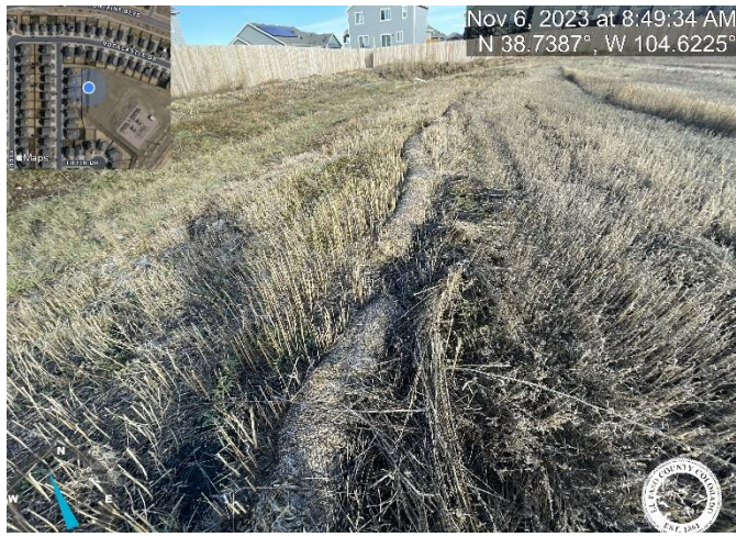
Photo 17: Substation Swale 2: Remove temporary control measures from swale.
