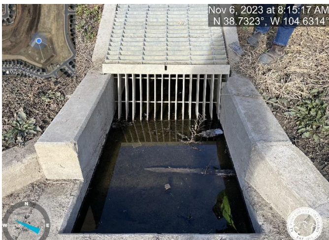
Photo 7: Remove sediment and debris from outlet structure micropool.
