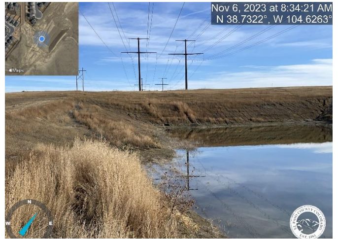
Photo 2: Implement missing Gravel Access Road. Reference sheet C5.2 of the Final Grading and Erosion Control Plans.
