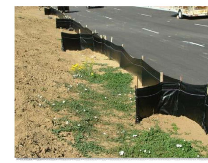
Photograph SF-2. When silt fence is not installed along the contour, a "J-hook" installation may be appropriate to ensure that the BMP does not create concentrated flow parallel to the silt fence. Photo courtesy of Tom Gore.
