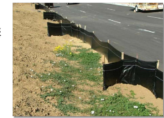
Photograph SF-2. When silt fence is not installed along the contour, a "J-hook" installation may be appropriate to ensure that the BMP does not create concentrated flow parallel to the silt fence. Photo courtesy of Tom Gere.
