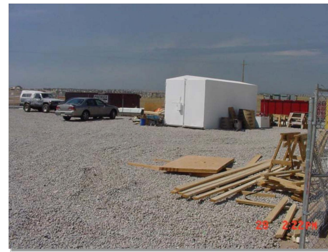
Photograph SSA-1. Example of a staging area with a gravel surface to prevent mud tracking and reduce runoff. Photo courtesy of Douglas County.
