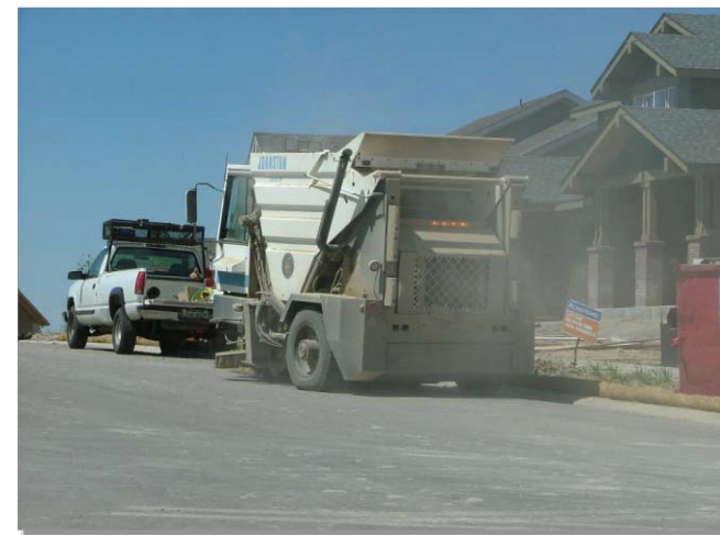
Photograph SS-1. A street sweeper removes sediment and potential pollutants along the curb line at a construction site. Photo courtesy of Tom Gore.
