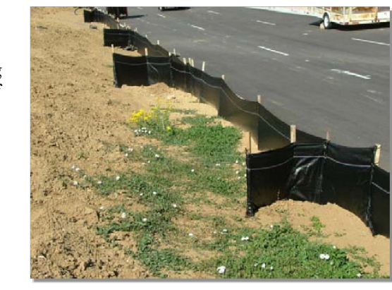
Photograph SF-2. When silt fence is not installed along the contour, a "J-hook" installation may be appropriate to ensure that the BMP does not create concentrated flow parallel to the silt fence. Photo courtesy of Tom Gere.
