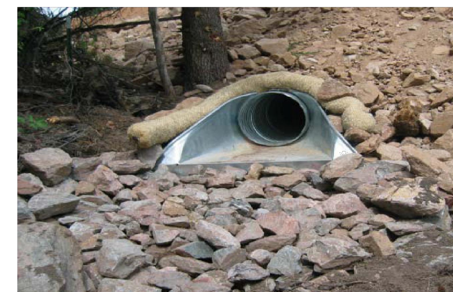
Photograph TOP-1. Riprap outlet protection.
