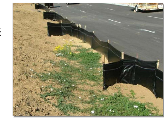
Photograph SF-2. When silt fence is not installed along the contour, a "J-hook" installation may be appropriate to ensure that the BMP does not create concentrated flow parallel to the silt fence. Photo courtesy of Tom Gere.
