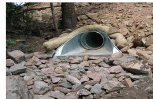
Photograph TOP-1. Riprap outlet protection.
