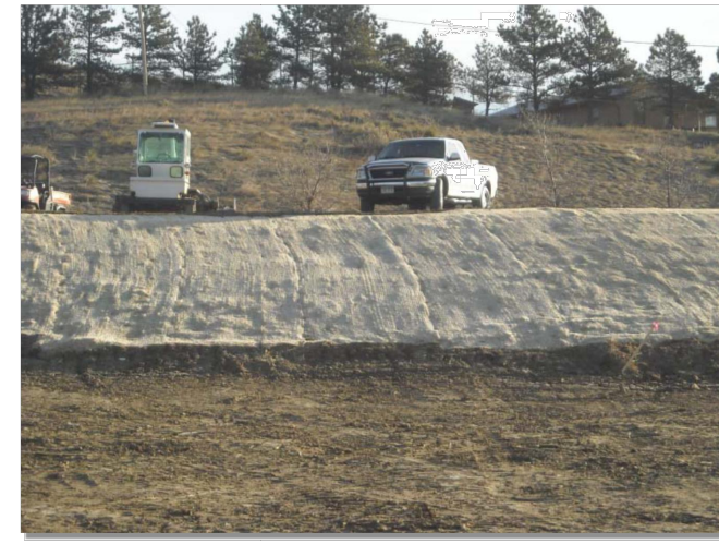
Photograph RECP-1. Erosion control blanket protecting the slope from erosion and providing favorable conditions for revegetation.
