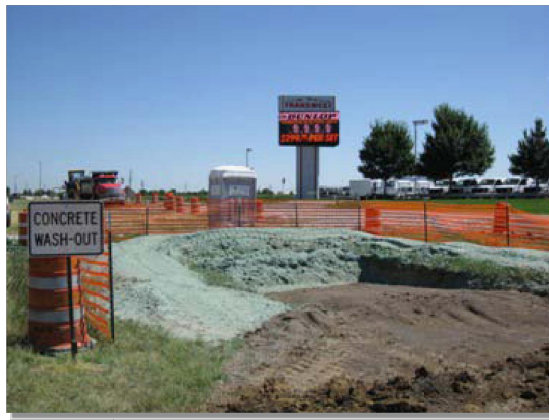
Photograph CWA-3. Earthen concrete washout. Photo courtesy of CDOT.
