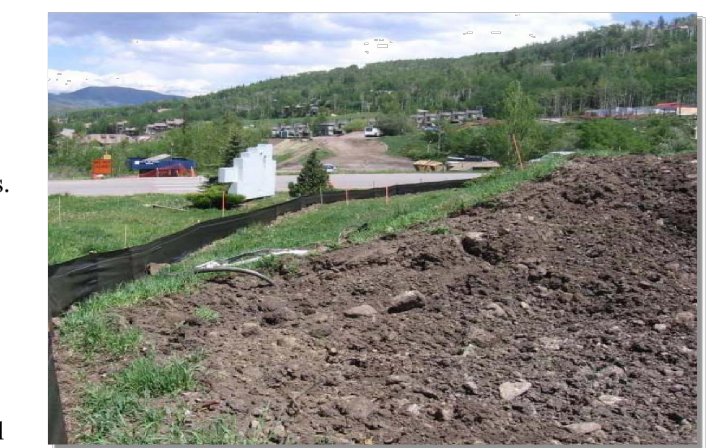
Photograph SP-1. A topsoil stockpile that has been partially revegetated and is protected by silt fence perimeter control.
