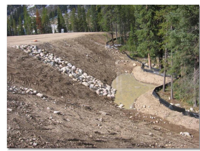
Photograph SB-1. Sediment basin at the toe of a slope. Photo courtesy of WWI.
