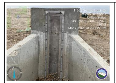
Photo 1: Well screen not installed per spec. (Figure OS-5) Page 5 of CD's
