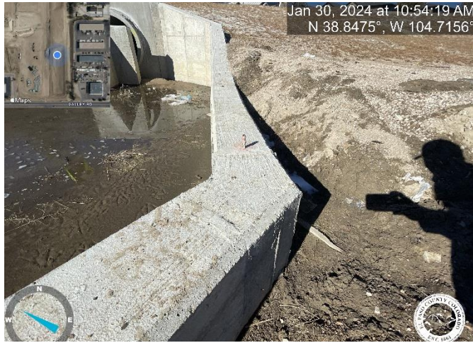
Photo 10: Remove exposed rebar from forebay B1.
