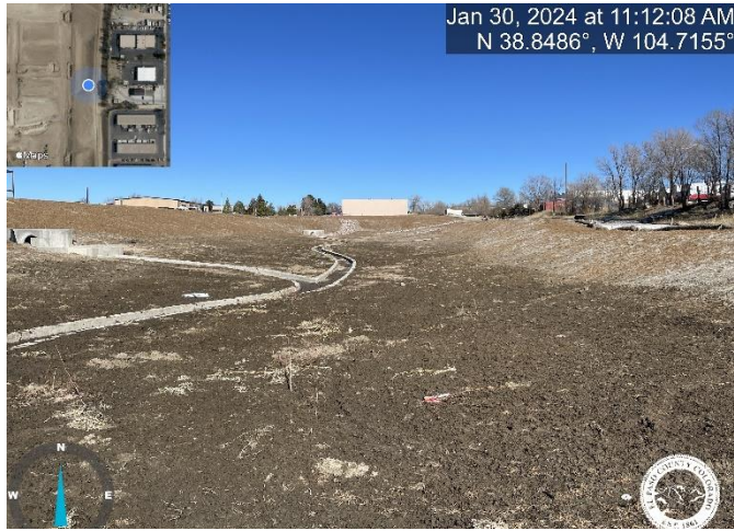
Photo17: Pond A: Fine grade Pond bottom to match the approved grade.
