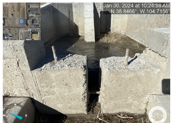
Photo 4: Pond B: Remove exposed rebar from forebay B2.
