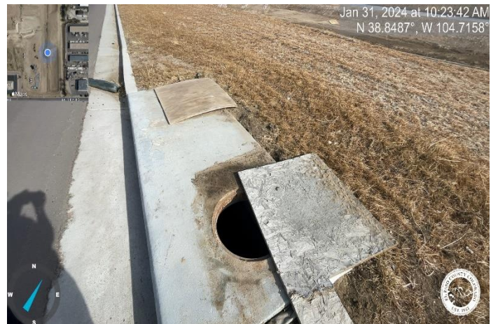
Photo 24: Inlet at STA 12+65.01: Install manhole lid.
