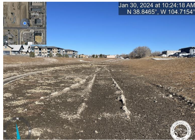
Photo 1: Pond B: Fine grade Pond bottom to match the approved grade.
