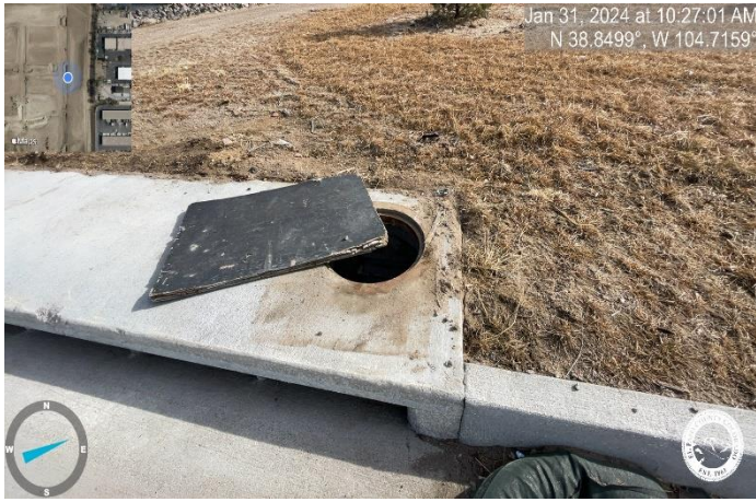
Photo 25: Inlet at STA 12+12.45: Install manhole lid.
