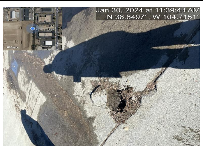
Photo 2: Approximately STA 14+05: Repair chipped concrete.
