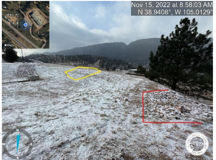
Photo 6: West detention pond; Emergency overflow path was not installed at proper location. Yellow box indicates the approximate location provided on Sheet C2.9 of the Erosion Control Plans, and the red box indicated the current installed location.
