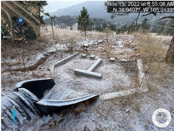
Photo 5: Remove sediment and debris from the forebay and riprap at STA 2+70.10
