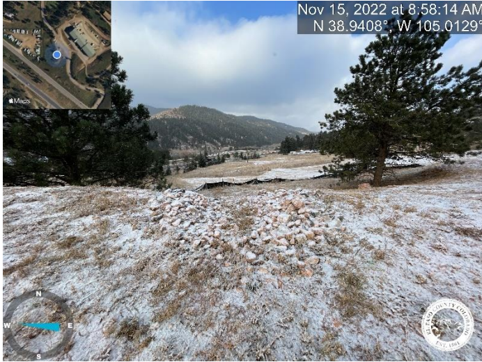
Photo 7: West detention pond; Emergency overflow path is not installed per detail. Provided detail on Sheet C2.9 shows that the path should measure 18' at the base.
