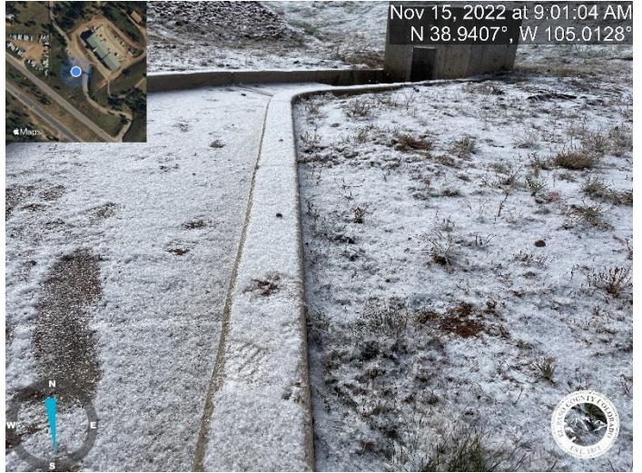
Photo 8: West extended detention pond; Raise pond bottom to top of trickle channel curb with a 3% slope towards trickle channel for positive drainage.
