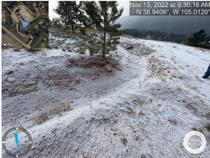
Photo 14: Fine grade ditch to promote positive drainage near STA 0+20.
