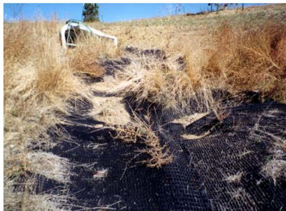
**Photograph 9-28.** Pipe outfalls are recommended over rundowns due to the high failure rate of rundowns.
