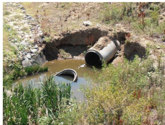
**Photograph 9-29.** Pipe end failure resulting in loss of the flared end section
