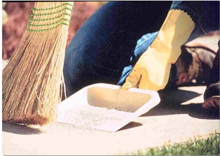
Photograph GH-1. Use dry clean-up methods to remove spilled materials. Photo courtesy of Colorado Nonpoint Source Program.
