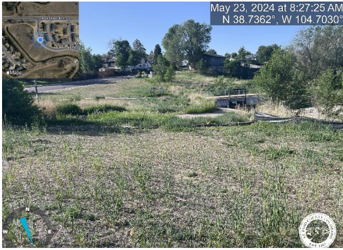
Photo 5: Remove all temporary control measures (silt fence, straw wattle and rock socks) site wide.
