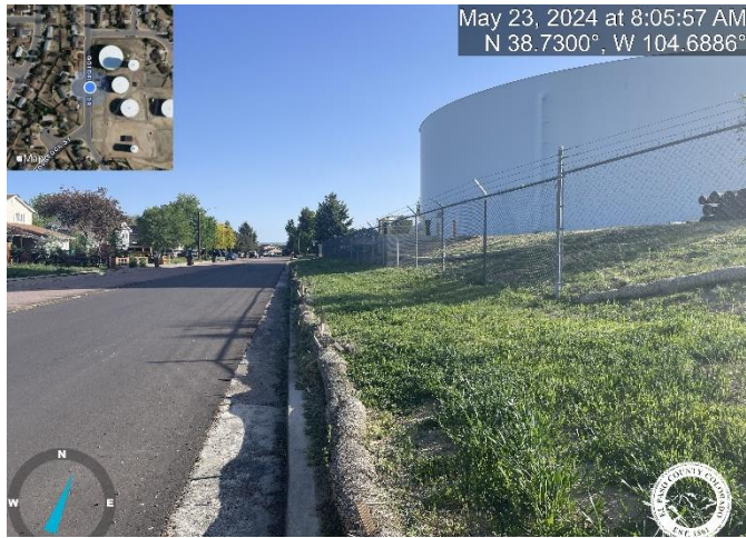
Photo 1: Remove all temporary control measures (silt fence, straw wattle and rock socks) site wide.
