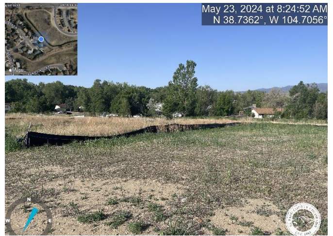
Photo 4: Remove all temporary control measures (silt fence, straw wattle and rock socks) site wide.
