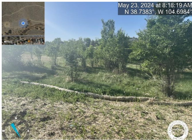
Photo 3: Remove all temporary control measures (silt fence, straw wattle and rock socks) site wide.
